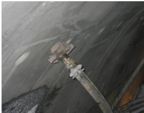
Grout hose fixed to socket on inner surface of tunnel segment.
