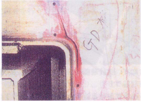
Photo 9 Fatigue crack at corner cut of girder end 1)
