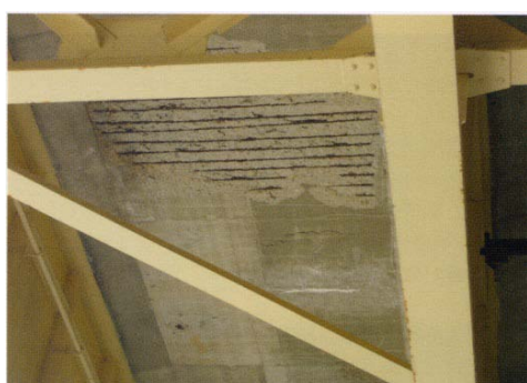
Photo 13 Replacement of concrete deck slab 1)
