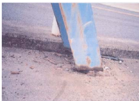
Photo 8 Brokenness of flange in a diagonal member in a truss bridge 1)
