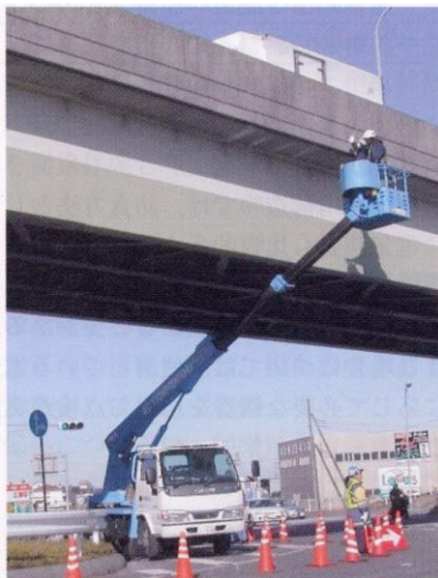
Photo 1 Inspection vehicle 1) (for high position work)
