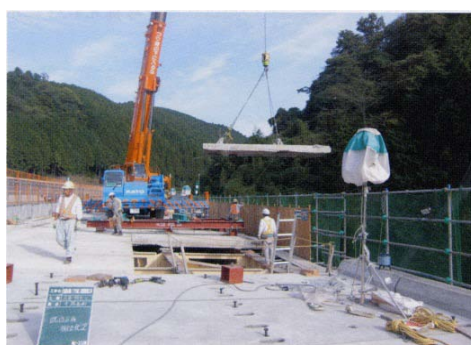
Photo 13 Replacement of concrete deck slab 1)
