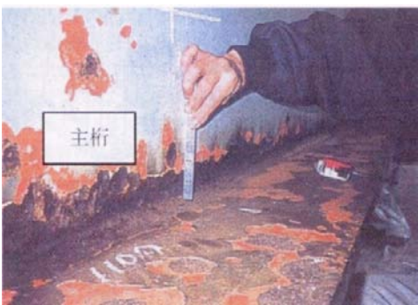
Photo 7 Corrosion at fillet welding between web and lower flange 1)
