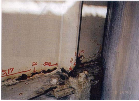
Photo 6 Corrosion at girder end 1)
