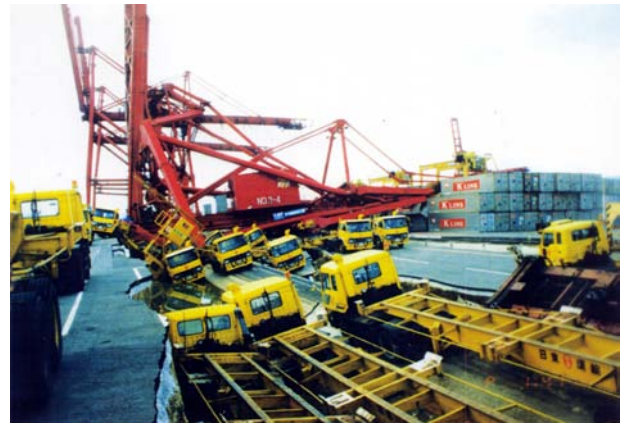
Photo 2 Damage on the wharf
