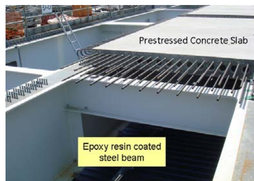
Fig.9 Upper Structure of Wharf Type Runway
