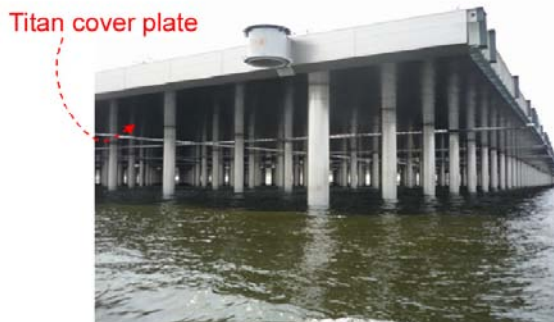
Fig.8 Lower Structure of Wharf Type Runway
