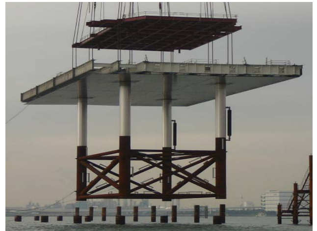
Photo 6 Installation of jacket part
