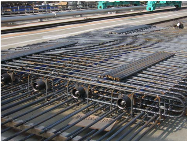
Photo 2 Steel arrangement at slab panel
