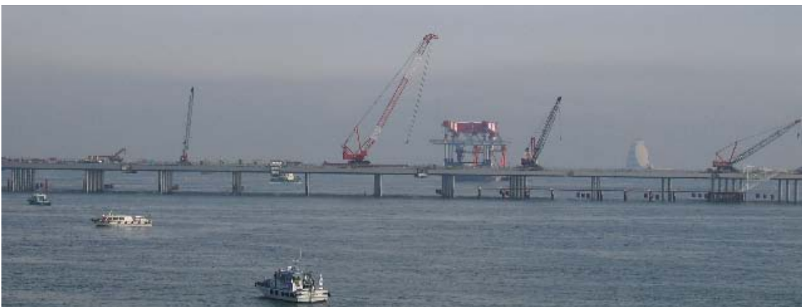
Photo 1 Construction site in 2008
