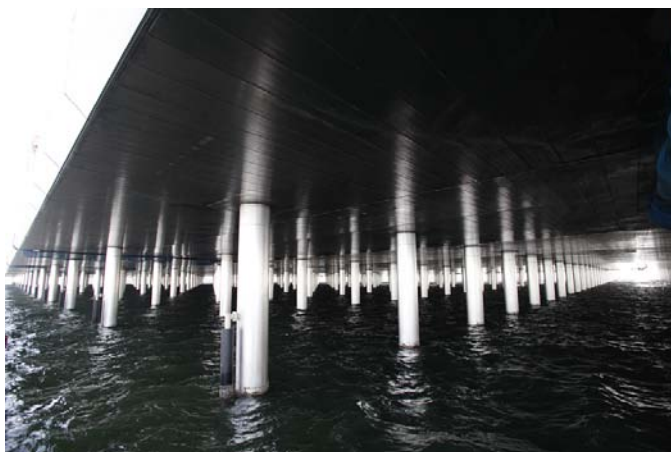
Photo 8 View of piles covered by stainless steel
