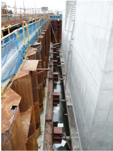
Photo 11 Joint of the piles
