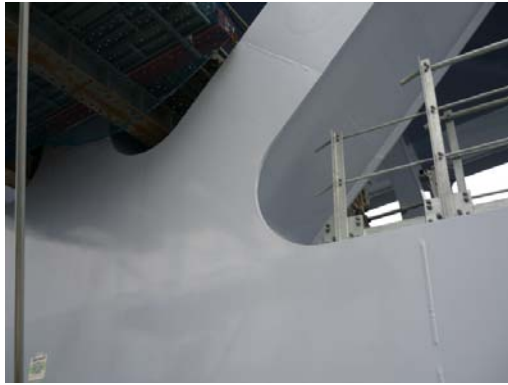
Photo 14 Truss joint part by welding
