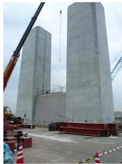
Photo 13 Completed main pier
