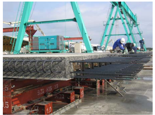
Photo 3 Fabricated slab panel
